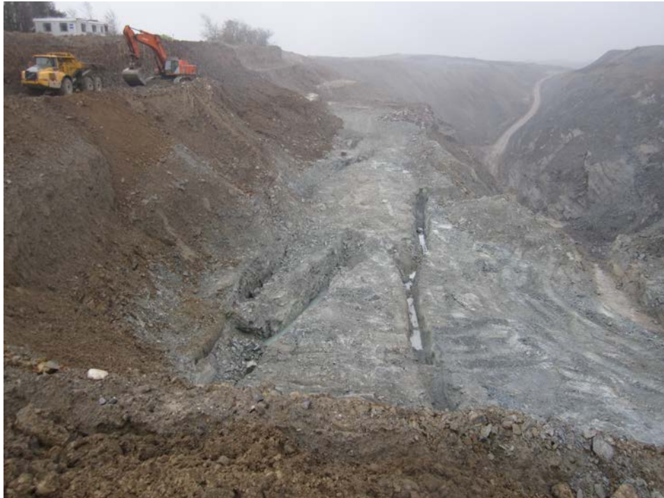
FIGURE 6. KEARNEY PIT LOOKING SOUTH AFTER EXTRACTION OF VEINS
