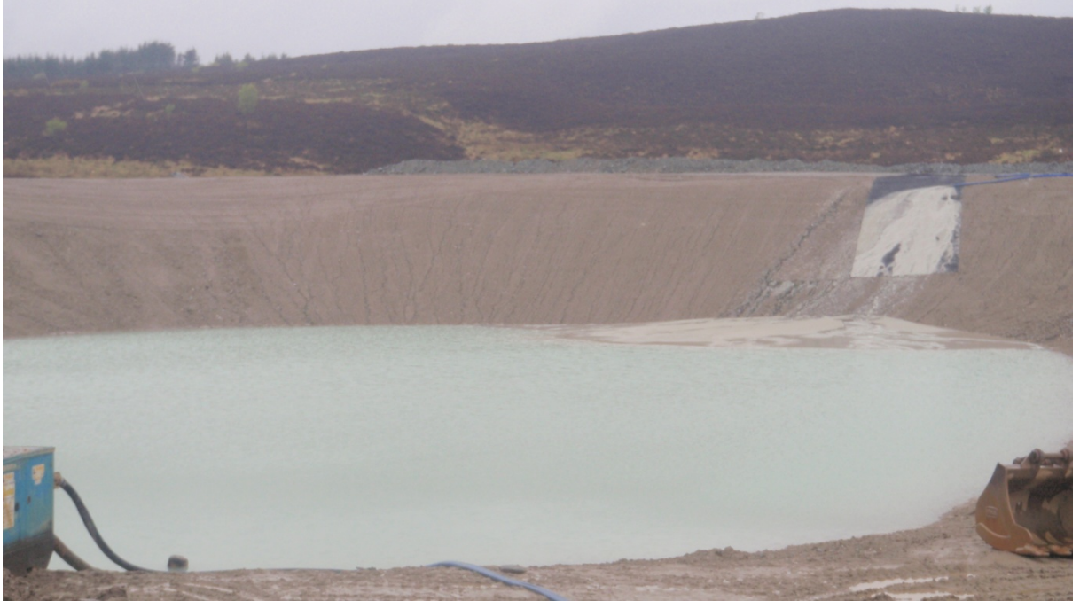
FIGURE 28. TAILINGS PASTE CELL BEING FILLED
